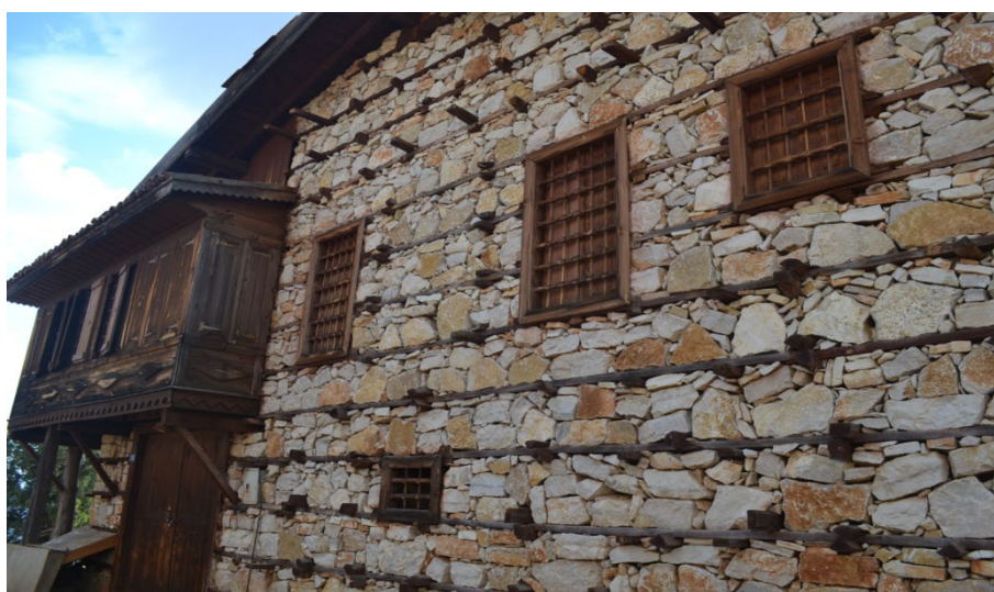
Figure 2. The wall technique unique to the locality (09.29.2015, Sarihacilar Neighborhood, Akseki).
